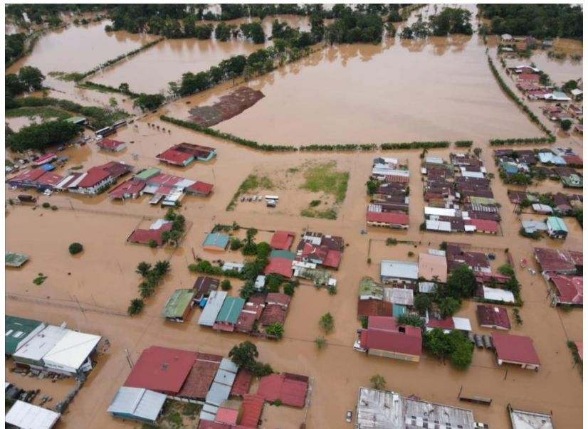
Areas flooded in Limon – Source – National Emergency Commission
