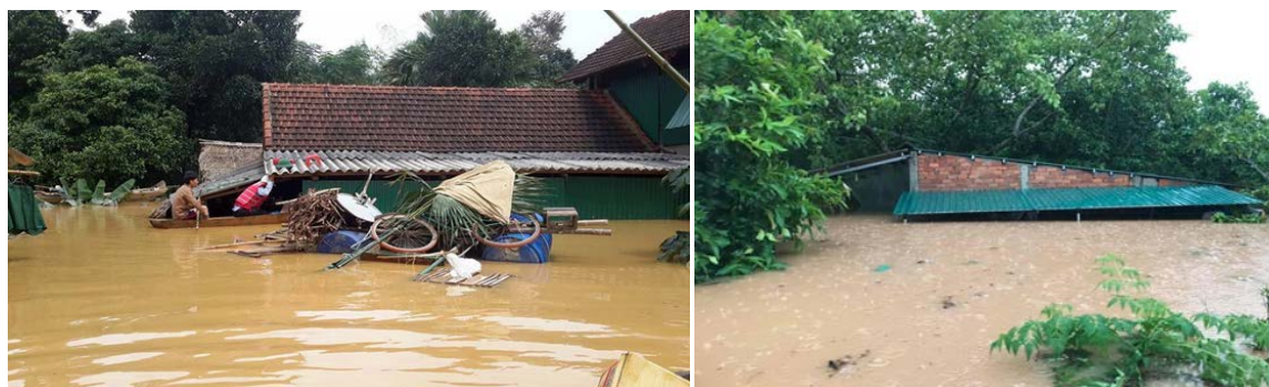
Floods affected houses in Quang Tri province. (Photo: VNRC)
