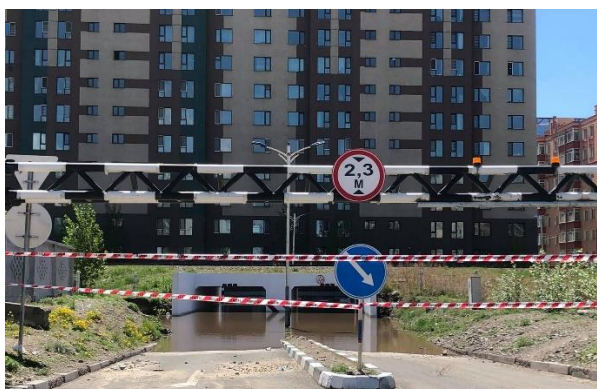
Flooded tunnel in the capital. Photo: MRCS.
