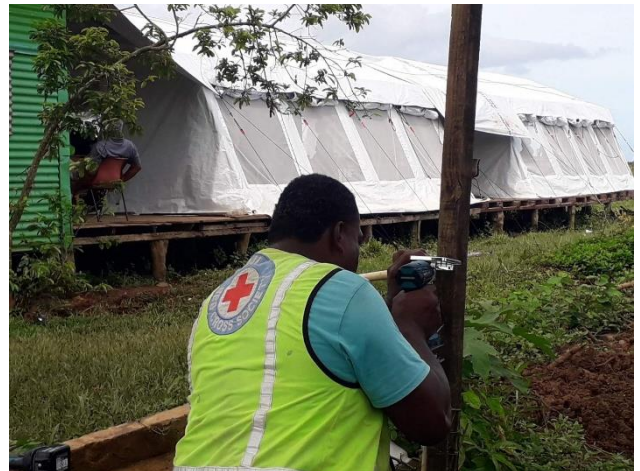
Installation of handwashing station at a school, Macuata (Photo: FRCS)
