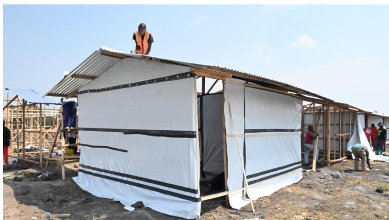
Shelter construction by DRC RC volunteers. ©IFRC
