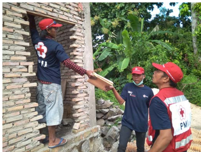
SIBAT members supporting the permanent shelter construction in Lampung. (Photo: PMI)
