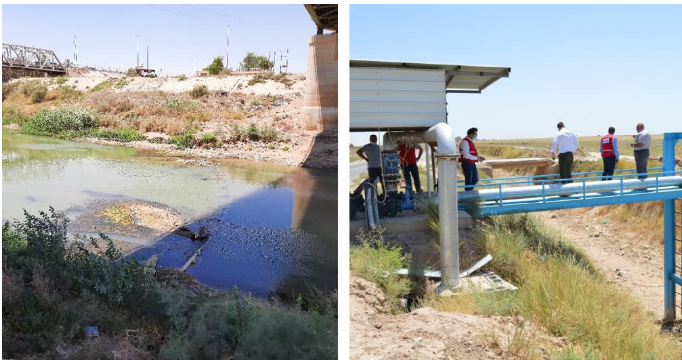
Figure 5: Diyala river and its tributaries in 2021 after depleted the water. Photo by: IRCS
