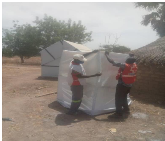
Volunteers building latrines in Mayo Danay. © CRC
