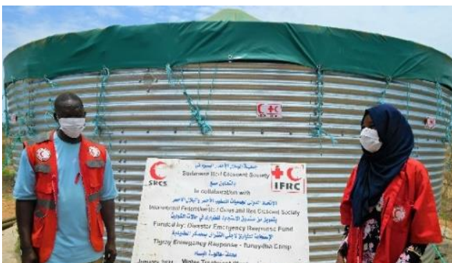
Sudan, Gedaref, El Tunaydba refugee camp. The water treatment plant in Tunaydba produces 265,000 litres per day. The SRCS dispatches close to 15 trucks of water per day, and they deliver 250,000 litres to refugee families within the camp and 15'000 Litres to the host community. Rita Nyaga ©IFRC
