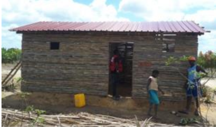
Figure 12: TRANSITIONAL SHELTER type 3—Floor: Stabilized soil, Walls: Bamboo external / earth internal, Roof: 0.4mm thick IBR sheets.
