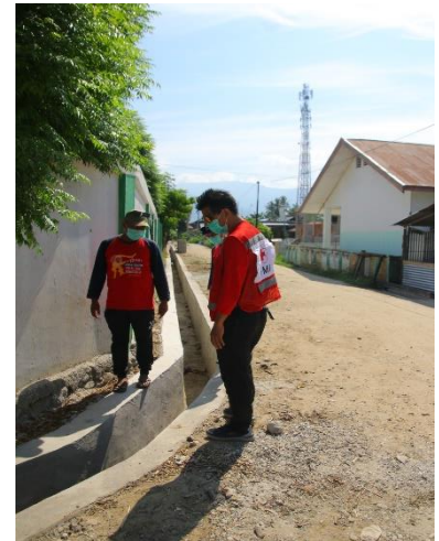
Site visit by PMI and CBAT before handover to the contractor.
