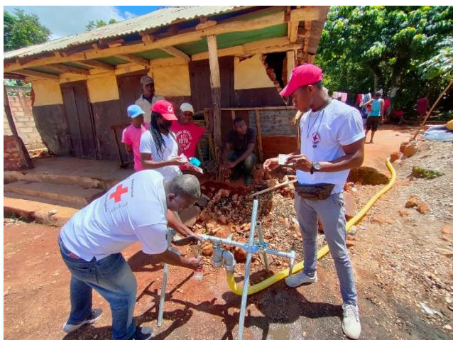
The Spanish Red Cross is supporting the HRCS to provide SETA units for water treatment and distribution. Source: Spanish Red Cross.
