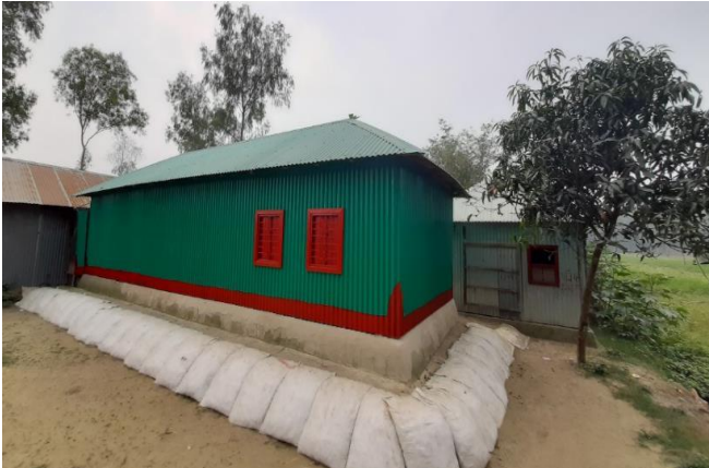
One of the flood-resilient shelters in the community. Beneficiaries constructed their shelter's considering recent years' flood level, Sirajganj (Photo: IFRC).
