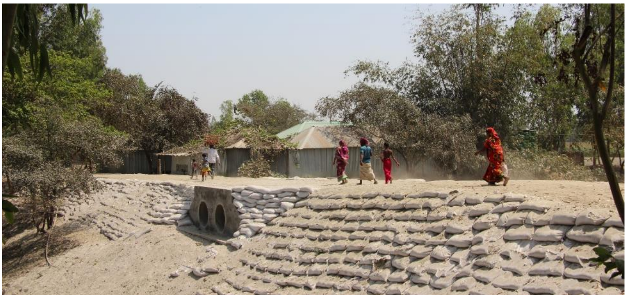
Earthen road in the community of Sirajganj; communication has been established between the communities via this road, even during floods. (Photo: BDRCS/IFRC)
