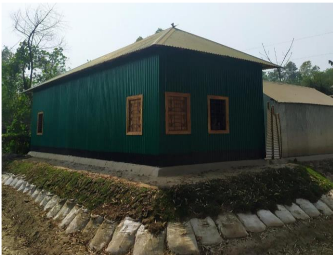
Beneficiaries constructed their flood resilient shelter by raising the plinth considering so that the shelters will not be submerged in the future. (Photo: BDRCS/IFRC)
