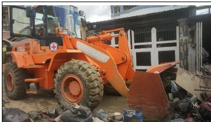
Clearing and flushing operations in Rodriguez Rizal. Photo: PRC.
