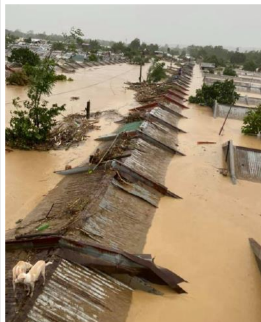
Flooding brought by Typhoon Vamco in Rodriguez Rizal. Photo: PRC
