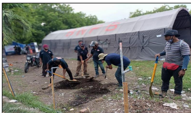
PMI Volunteers constructing Infiltration holes in Kantor Bupati Lama (Photo: PMI)
