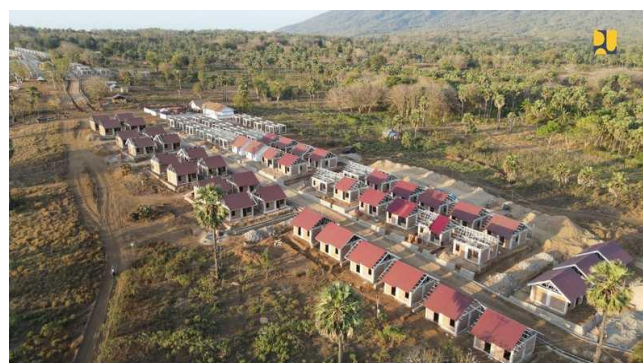
Construction Progress of the Relocation Sites in Lembata. (Photo: Investor.ID)
