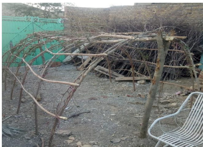
People using local materials to construct shelter. (Photo: PRCS)
