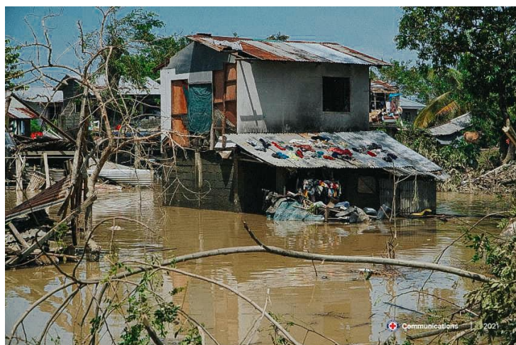
Flooding in La Union, Region I after the Severe Tropical Storm Kompasu (Maring). Photo: PRC
