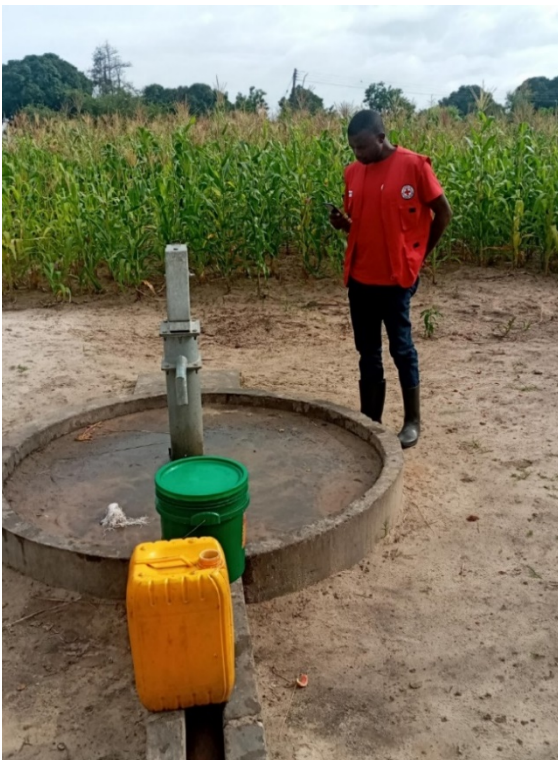
One of the water points rehabilitated in Kalabo
