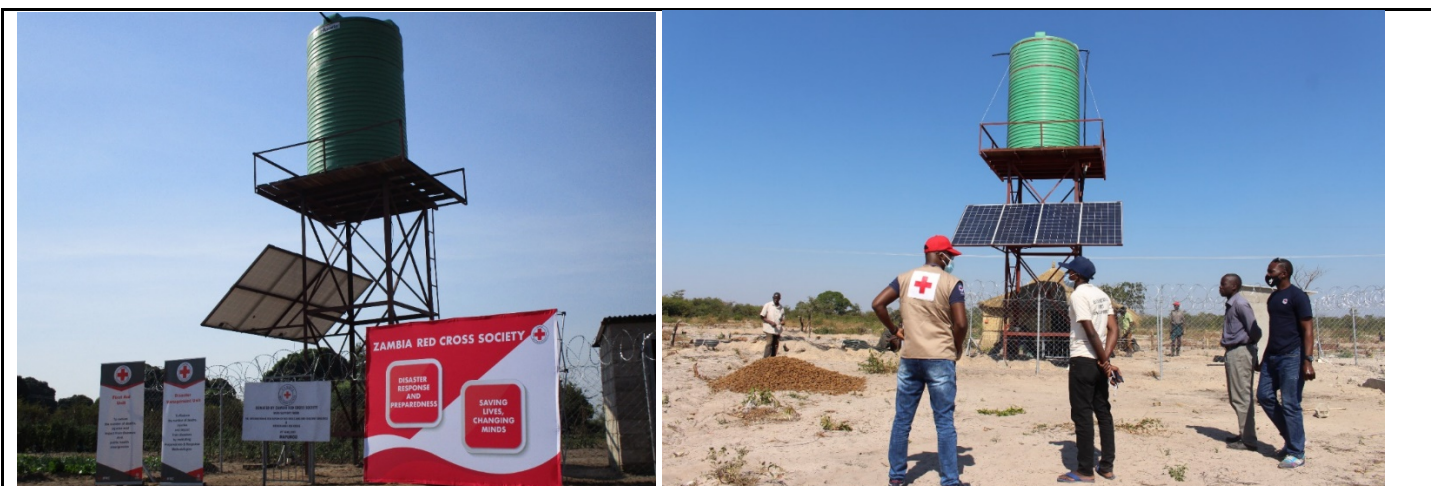
Figures above showing boreholes equipped with solar and tank for effective, sufficient and all year-round water supply
