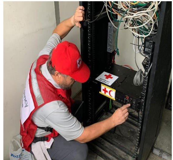
Installation of repeater at Levi Camp Perrin.
