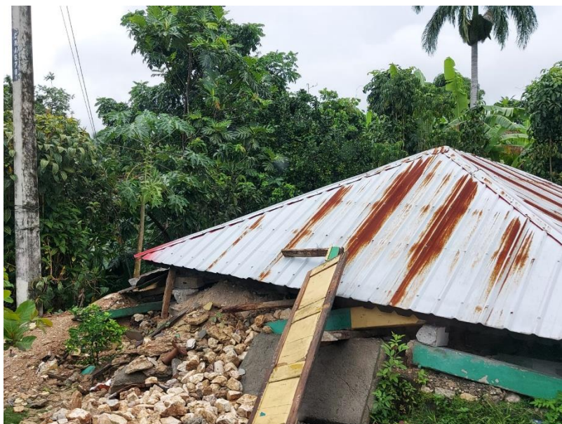
Collapsed house near Camp Perrin, Haiti, due to the 14 August earthquake.
