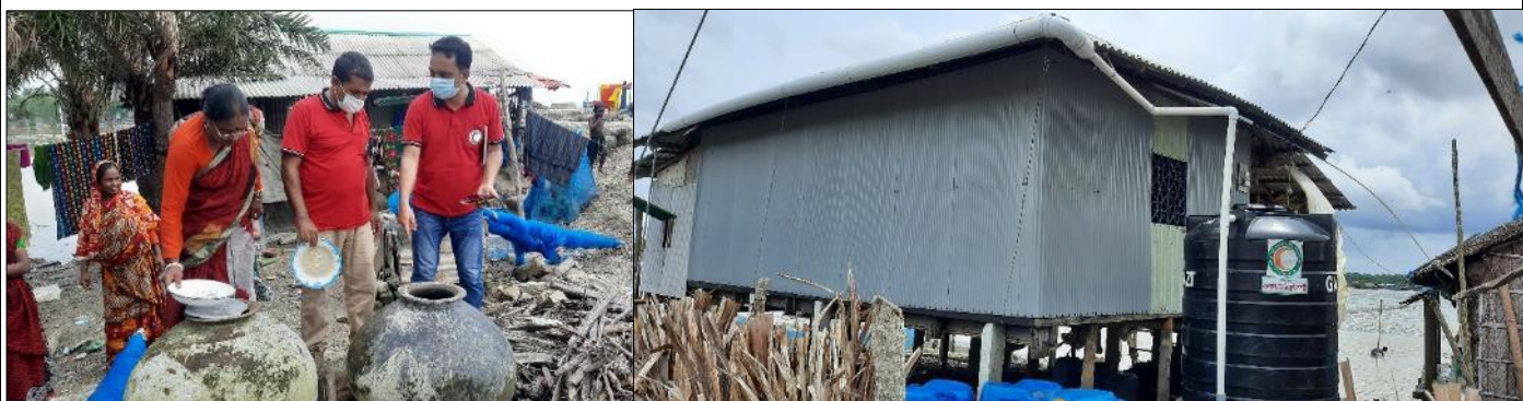
BDRCS consulting with community people regarding existing water consumption and storage practices (left) and considering the scarcity of safe drinking water, BDRCS installed rainwater harvesting system in the most cyclone-affected areas in Khulna (right). (Photos: IFRC)
