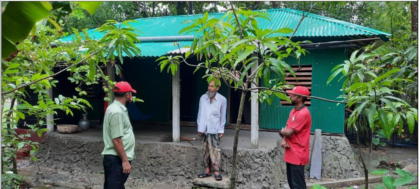
One of the reconstructed houses (with support from BDRCS) in Khulna. (Photo: IFRC)
