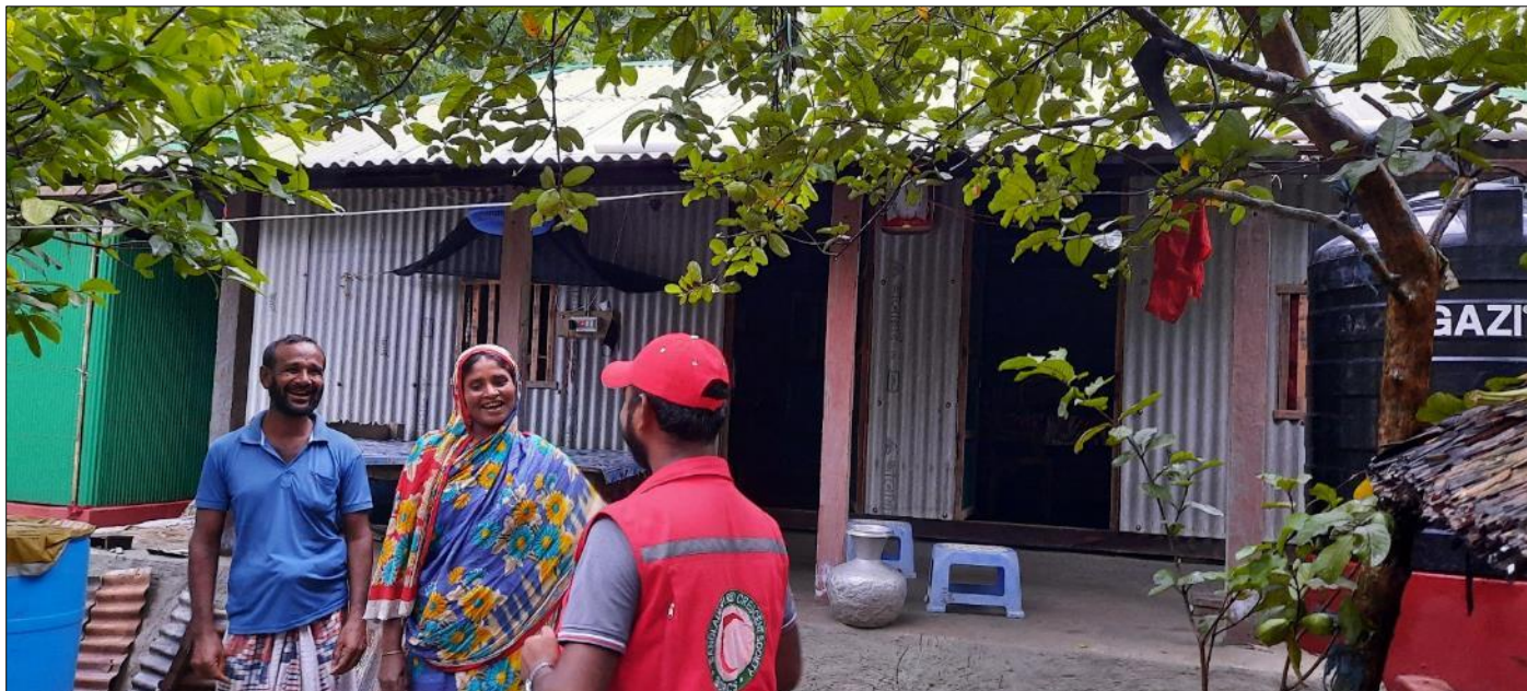
One of the beneficiaries completed shelter repair along with the rainwater harvesting unit and latrine installation in Khulna. (Photo: IFRC)
