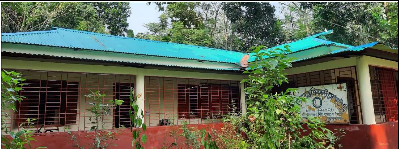
One of the repaired MCH centres. (Photo: IFRC)
