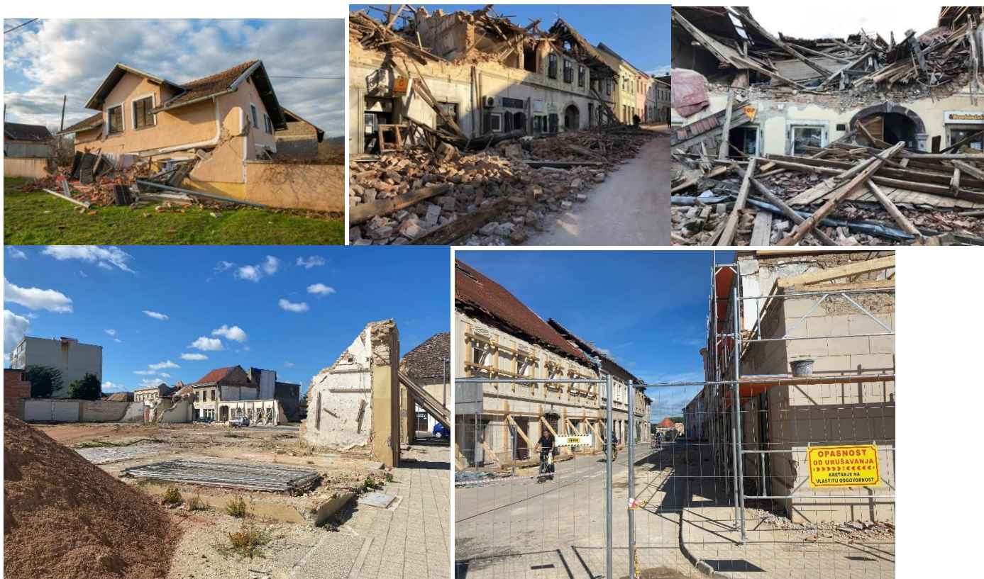
Photos by CRC: Photographs taken in the days and weeks following the earthquake on 29 December. There is still rubble and damage visible into late September as well as sites with cleaned streets from debris, removed demolished buildings and reconstruction works that started in June and July 2021
