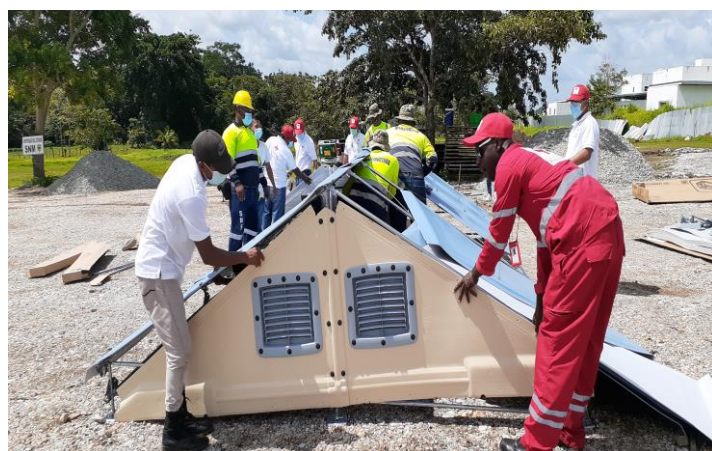
Installation of Shelters at ERM in Lajas Blancas, Panama. 2020
