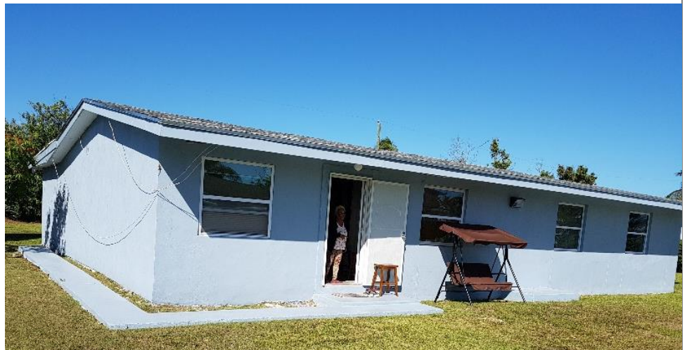
House repaired in Grand Bahama – February 2021 (Photo: BRCS).
