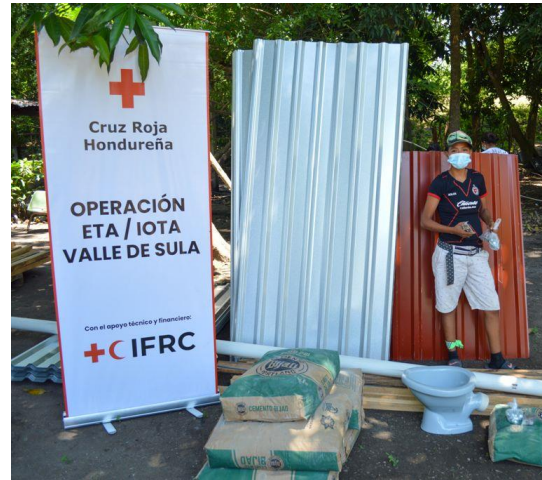
Delivery of materials for the construction of latrines in the community of La Protección, Choloma. September 2021. Source: HRC
