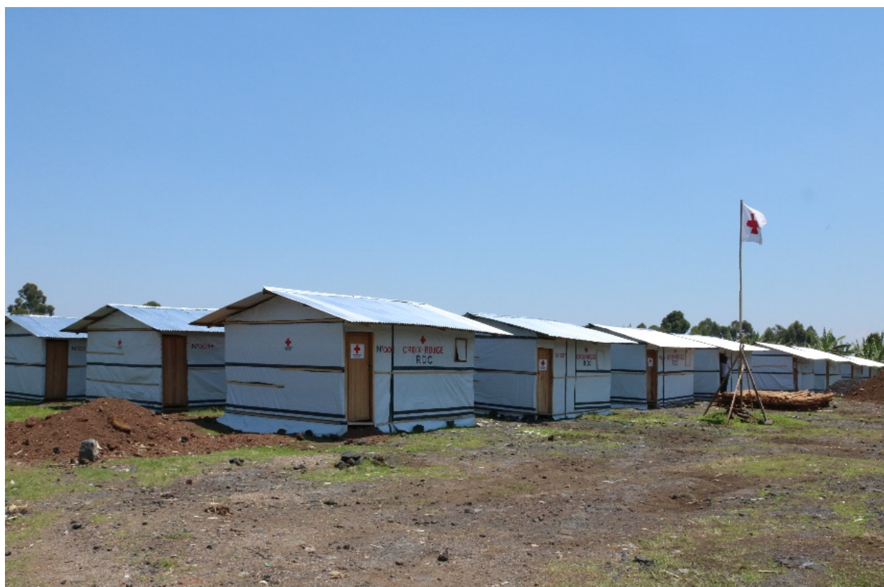
Shelter construction by DRC volunteers at temporary relocation site in Kibati, © DRC RC
