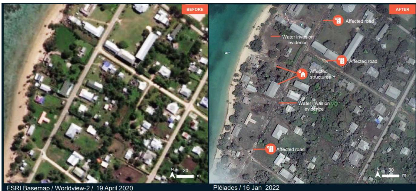
Before and after images of Lifuka village, Ha'apai Division, showing damage to buildings and structures. Source: United Nations Institute for Training and Research
