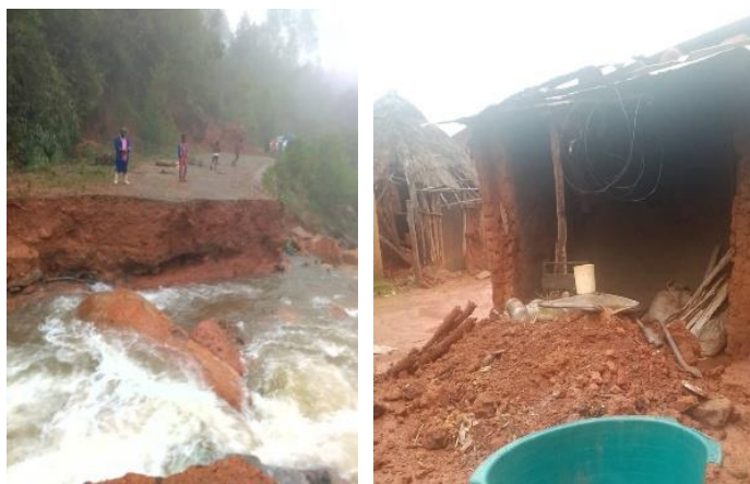
Figure 3: Shelter and Infrastructural Damage (above and below-right)
