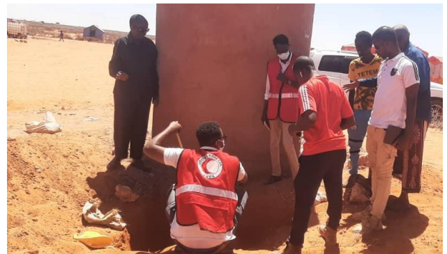
SRCS Team checking the construction of the 30 latrines in Jehdin as per the requirement of SRCS. This includes checking the measurement of latrine pits as the SRCS staff is doing in the picture.
