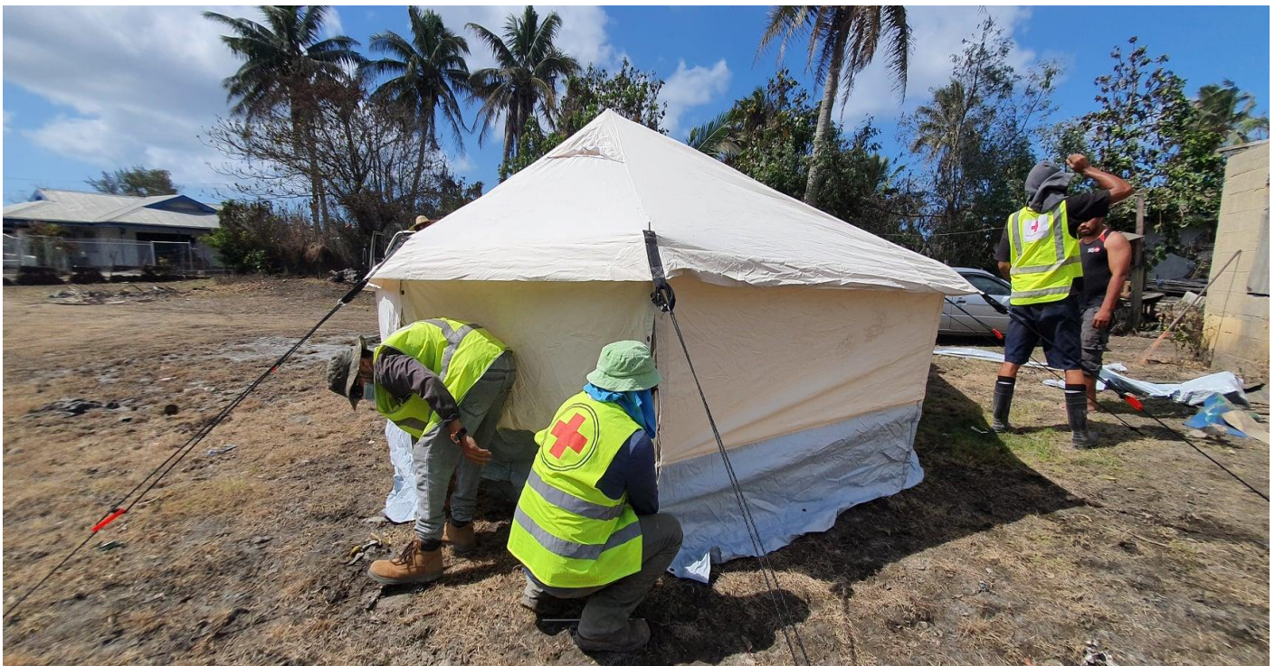
Tonga Red Cross Volunteers have assisted households in the worst affected areas on Tongatapu by distributing and erecting tents. Photo: TRCS
