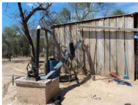
Tajamar – A different type of rainwater catchment system implemented in the area. Source: Municipality of Filadelfia
