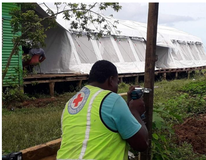
Installation of handwashing station at a school, Macuata. Photo: FRCS
