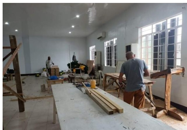
On-going rehabilitation of Catanduanes office. Photo: PRC
