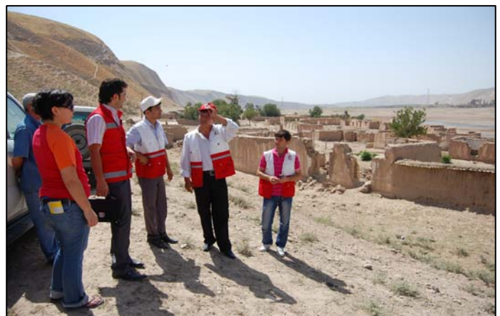
Village in Kulyab region, destroyed by floods. Photo: IFRC
