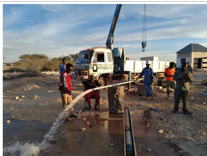
Rehabilitation of Gobsho Borehole
