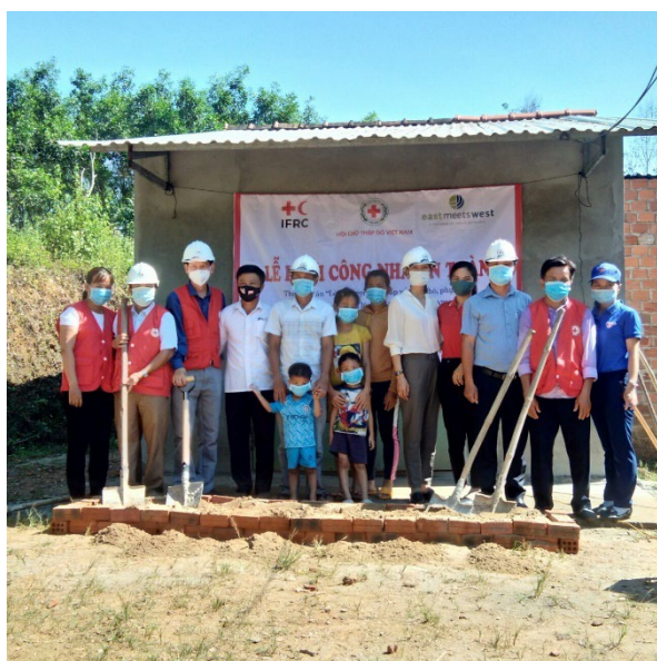
Flood resistant shelter construction commencement in Quang Nam (Photo: VNRC)
