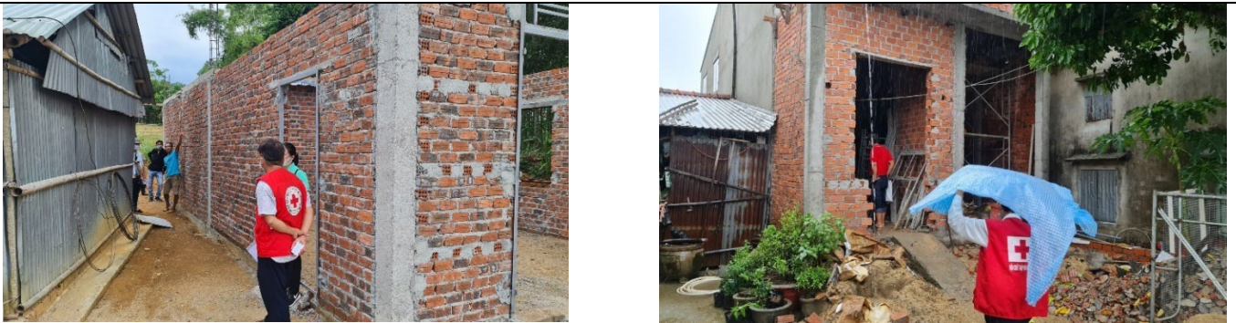
Shelter construction monitoring in Quang Nam province (Photo: VNRC)
