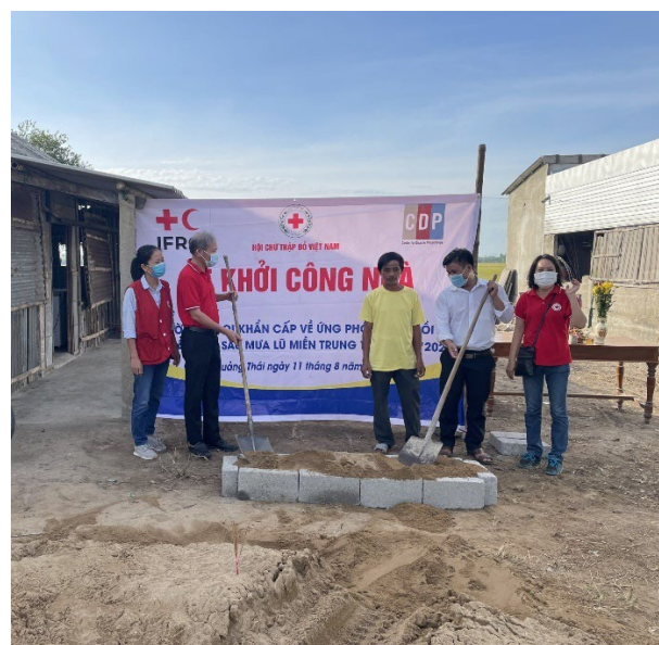
Commencement of flood resistant shelter construction in Hue (Photo: VNRC)
