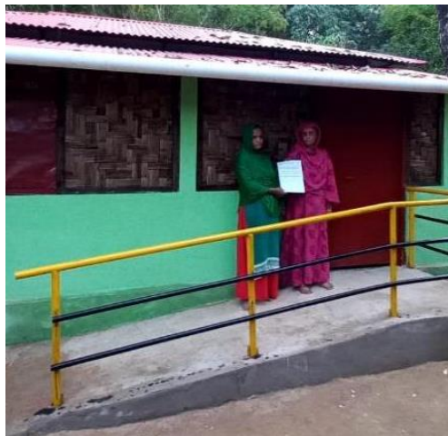
This shelter in the Ukhyia host community was modified in late 2021 with a ramp and railing to enable a person with disabilities to access the house. (Photo: BDRCS/American Red Cross)
