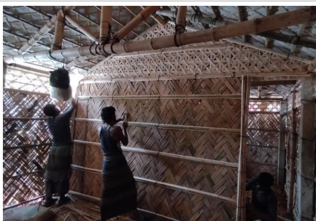
The 10 X 15-foot mid-term shelters in the camps feature a floor to ceiling partition which creates two compartments within the shelter, giving families some privacy and options on how to utilise the space. (Photo: IFRC)
