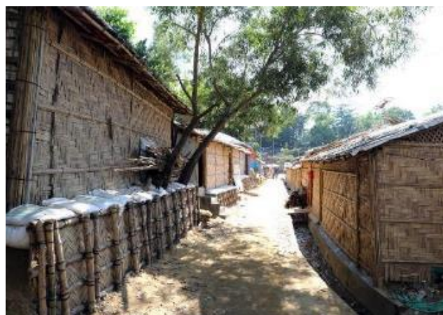
A mid-term shelter in Camp 12 with a guide wall to provide protection from flood or rainwater in the monsoon. (Photo: BDRCS)
