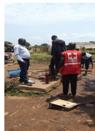
Figure 4: Monitoring of one of the rehabilitated boreholes
