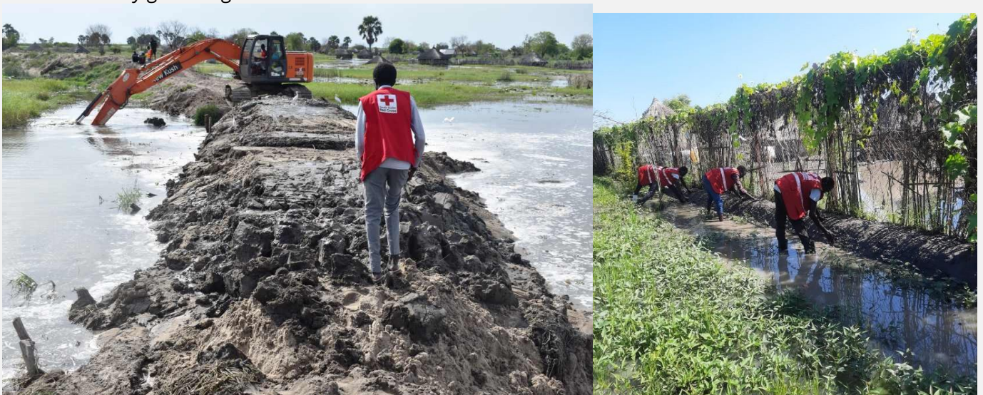
Figure 6: SSRC Supporting building of dykes
