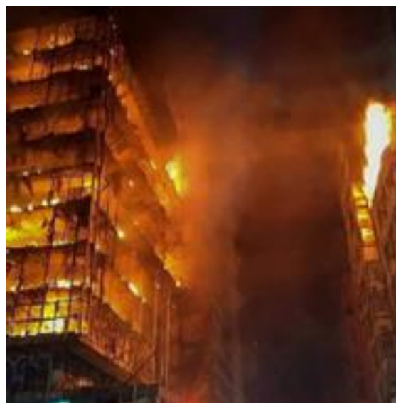
Fire break out in Hargeisa 01 April at 8pm
