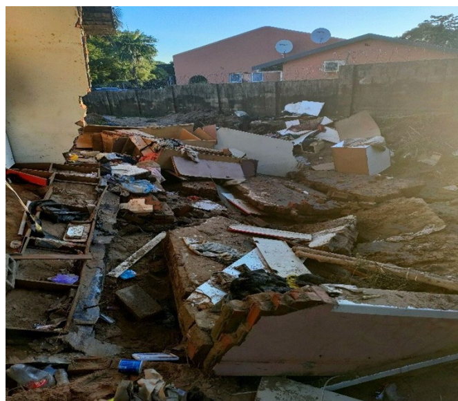
Figure 1: Floods damage in Tongaat area in eThekweni
