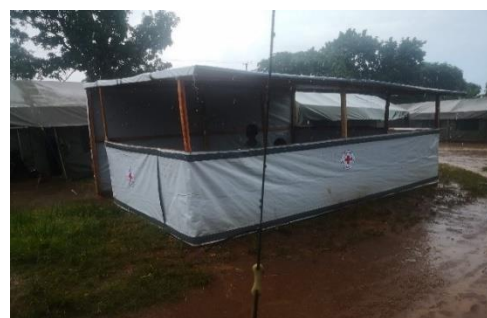
Temporary Kitchen shelter constructed in Ndola ©ZRCS
