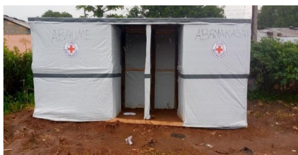
Temporary latrine constructed in Ndola Mapalo camp ©ZRCS
