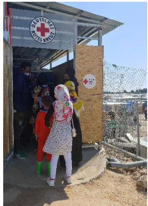
WASH facilities in Kara Tepe II Centre
