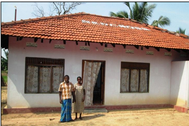
Mr Vellaisamy and wife in front of their completed house (photo: Kukan Sinniah, IFRC)
