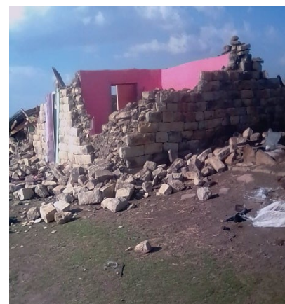
Figure 2: Destroyed house in Qacha's Nek ©LRCS
