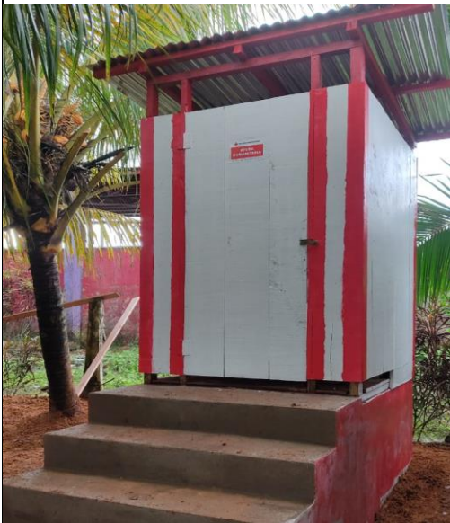
Construction of Community Latrine RACCN, December 2021. Source: NRC
