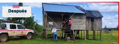
Reconstruction of house roof, Truskusirpi community, Waspam, May 17, 2022. Source: NRC
