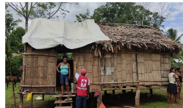
Family using a tarp donated by the project to cover the roof of a house, Cocal community, Waspam, May 12, 2022. Source: NRC
