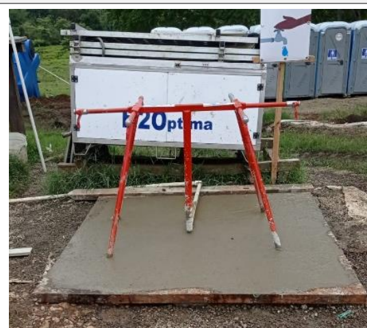
Hand-washing stations installed at different points in the ERM Lajas Blancas. Source: RCSP
