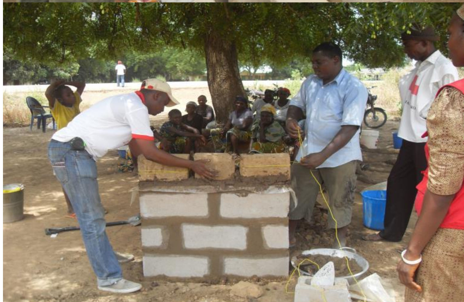
Flood resistant shelter building training in Ozahi (i) and Odogwu (ii)
