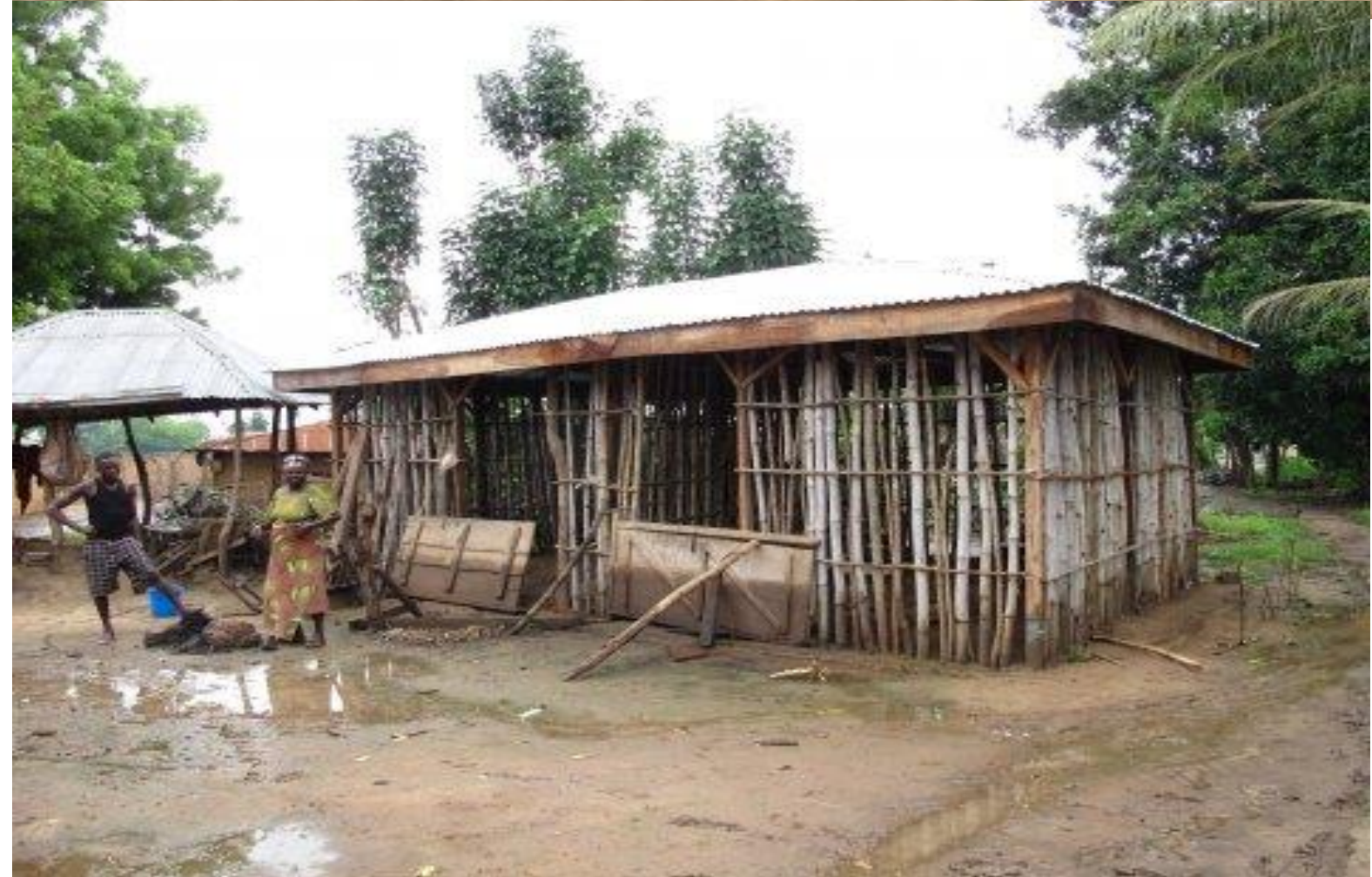
Early recovery shelters, which have been completed by beneficiaries in Mozum Ose (i) and Odogwu (ii)
