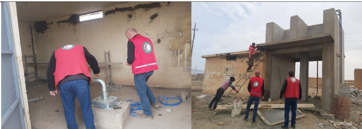
IRCS teams rehabilitate Water treatment plants/water points (Photo by: IRCS)
