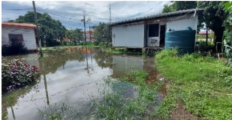
Flooding at the Tonga Red Cross National Headquarters in Tongatapu. (Photo: IFRC)
