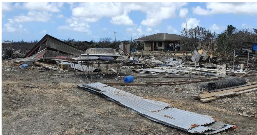
Following the volcano and tsunami, 167 homes were assessed as completely destroyed and a further 117 homes were assessed as being seriously damaged. (Photo: TRCS)
