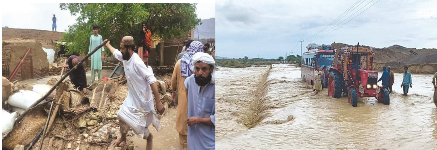
(Left) A view of damaged house due to recent rains in Karak; (Right) Roads washed away by floods in Hub, Balochistan (Photo Source: local media)
