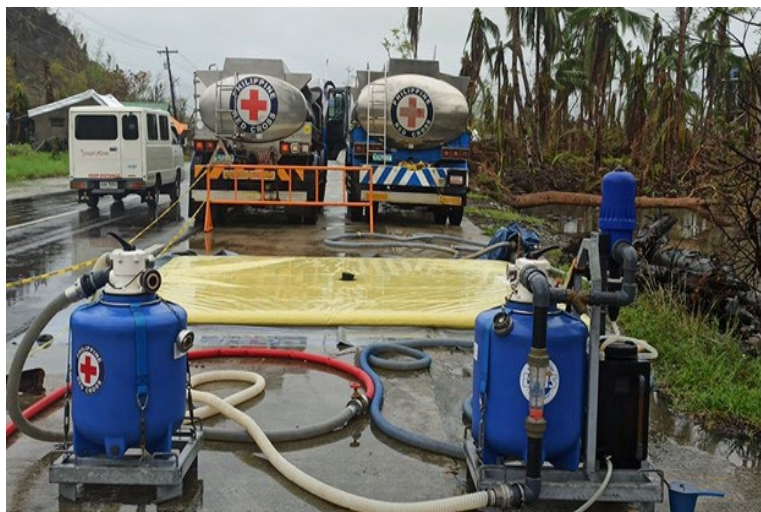
Water Production Site in Barangay Rizal, Surigao City (40,000 liters) per day. (Photo: PRC)
